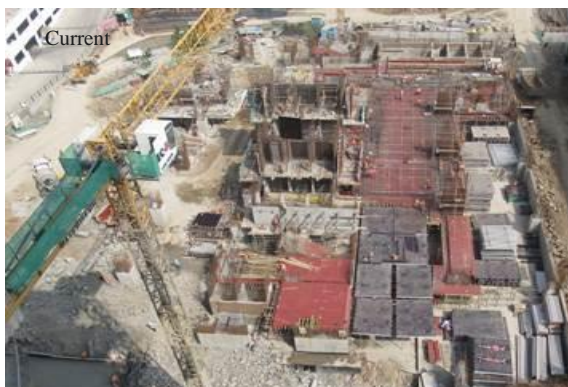
Building 5 – Podium level RCC work in progress
