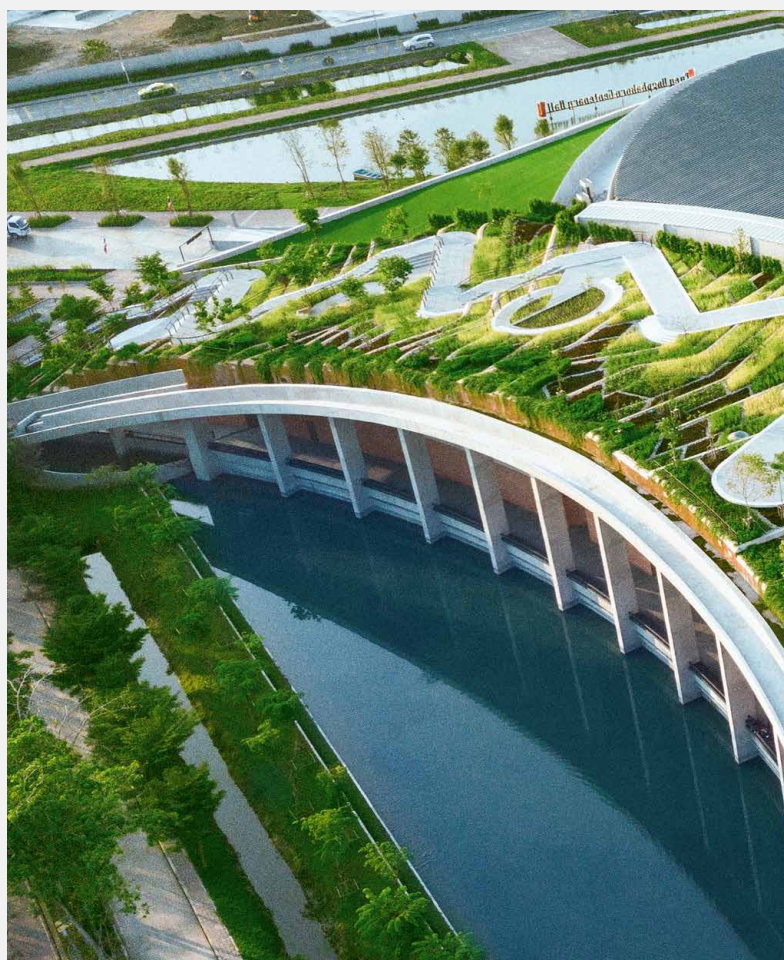
Thammasat University Rooftop Farm (TURF) Asia's largest rooftop farm, built with Firestone's UltraPly TPO 1.5mm – 20,000m 2 green roof in Thailand. >
